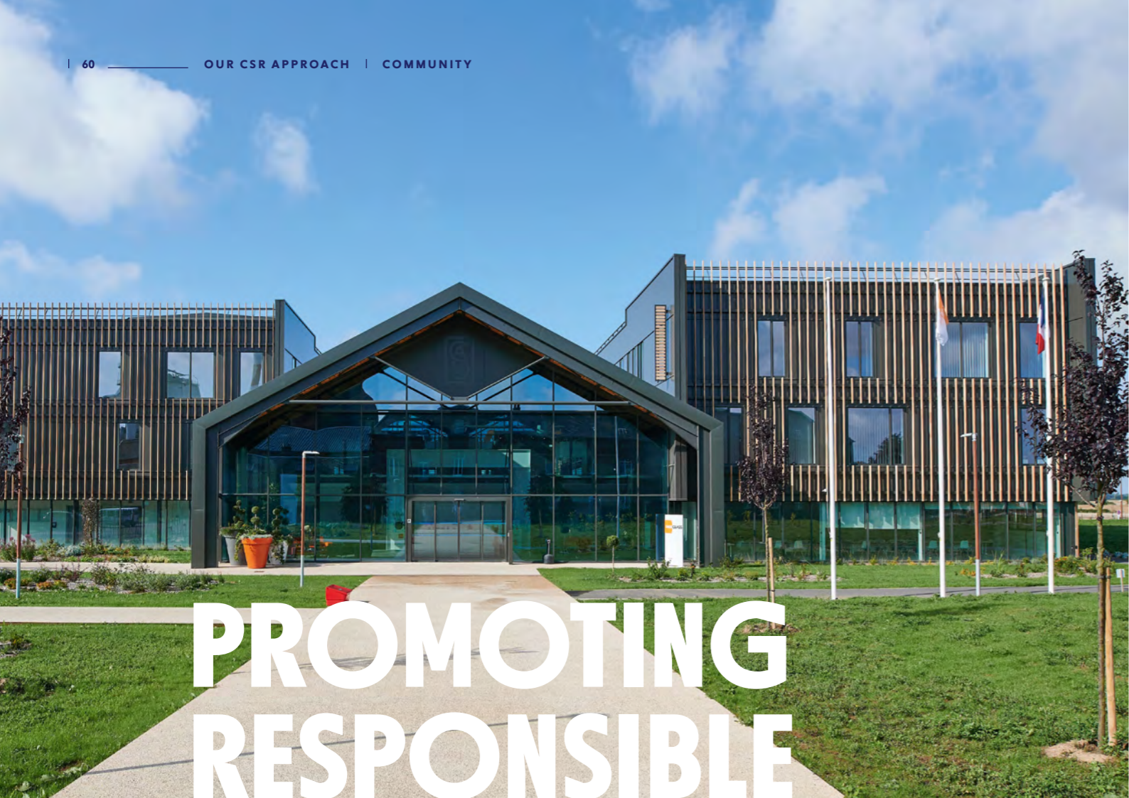
→ Group headquarters in Feuquières – France
