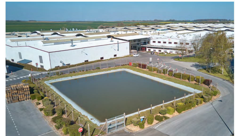
→ Rainwater collection tank – Feuquières – France
