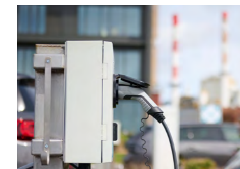
→ Charging station for hybrid vehicles – Feuquières – France
